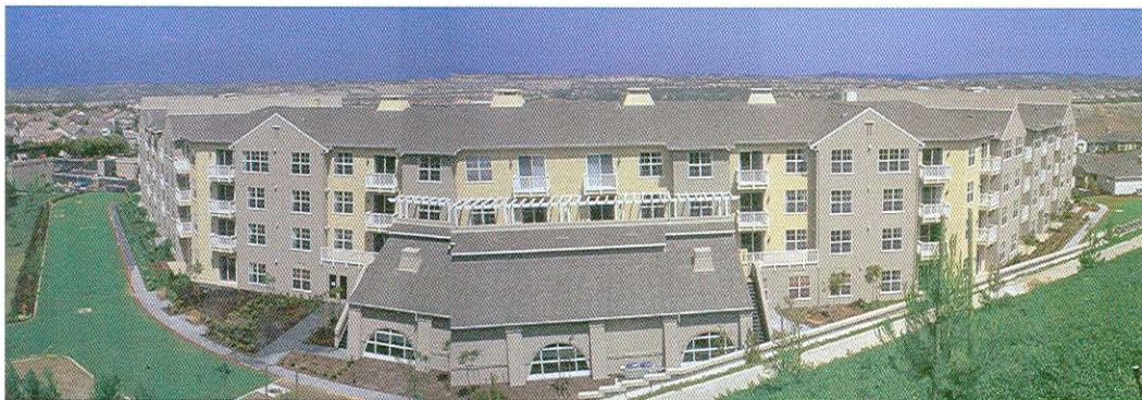
Photos courtesy of DPR Construction, Inc.
